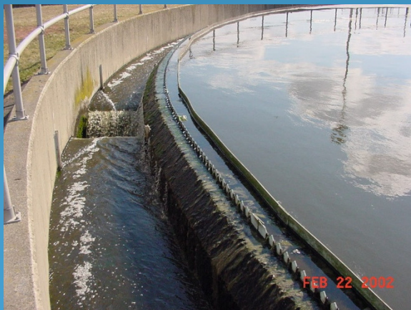
Typical V-Notch Weir
